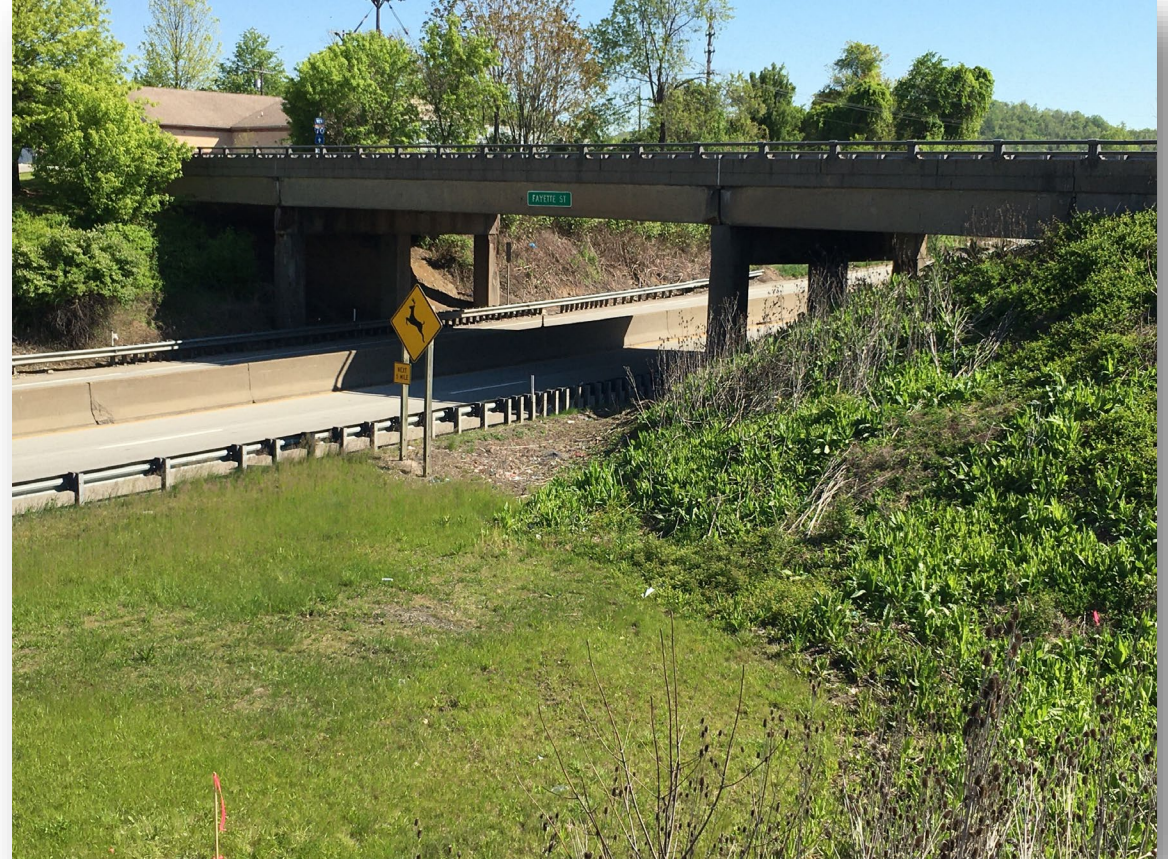
SR 3007 (Fayette Street) bridge over I-70
