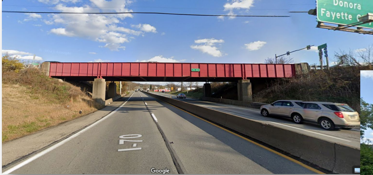
I-70 at SR 201 Bridge, Looking East
