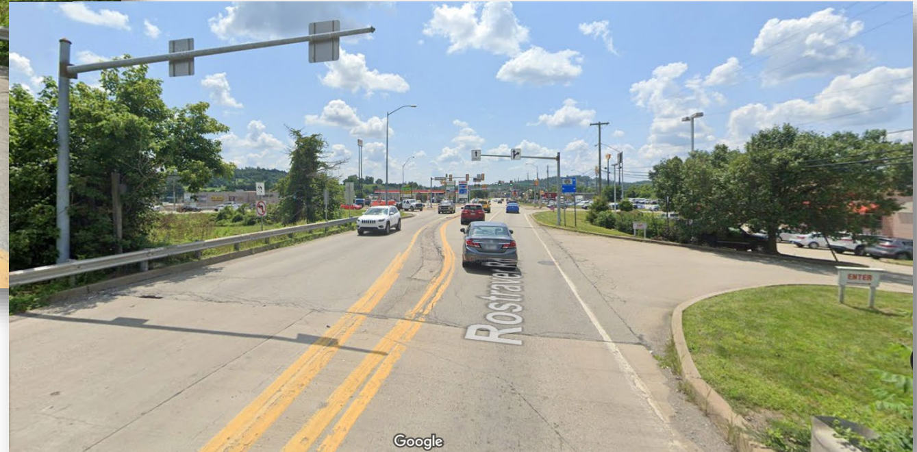
South End of SR 201 Bridge, Looking South
