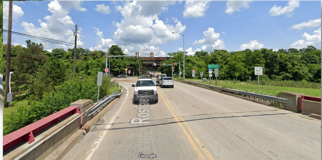
North End of SR 201 Bridge, Looking North
