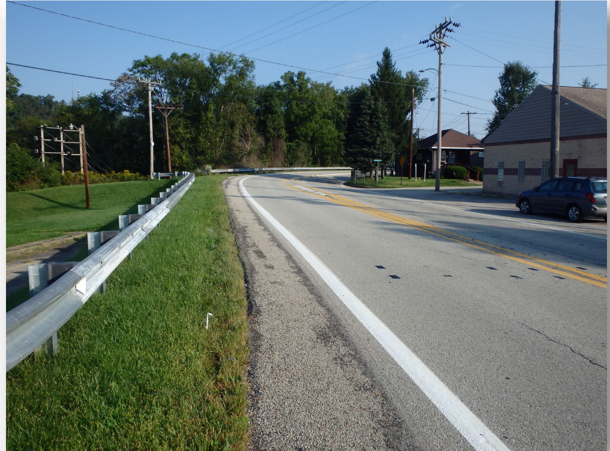
Stop Work, Looking North (Away From Bridge)
