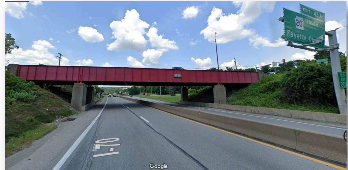
SR 201 (Rostraver Road) bridge over I-70
