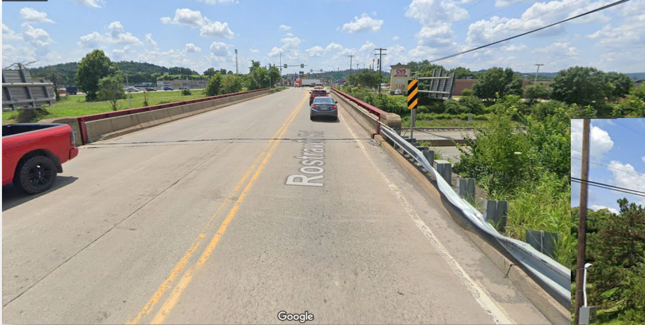
North End of SR 201 Bridge, Looking South
