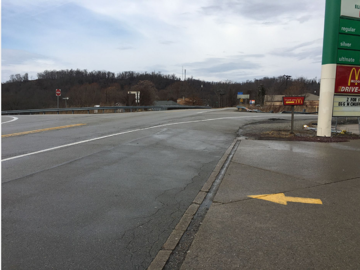
Start of Work, Looking North (Toward Bridge)
