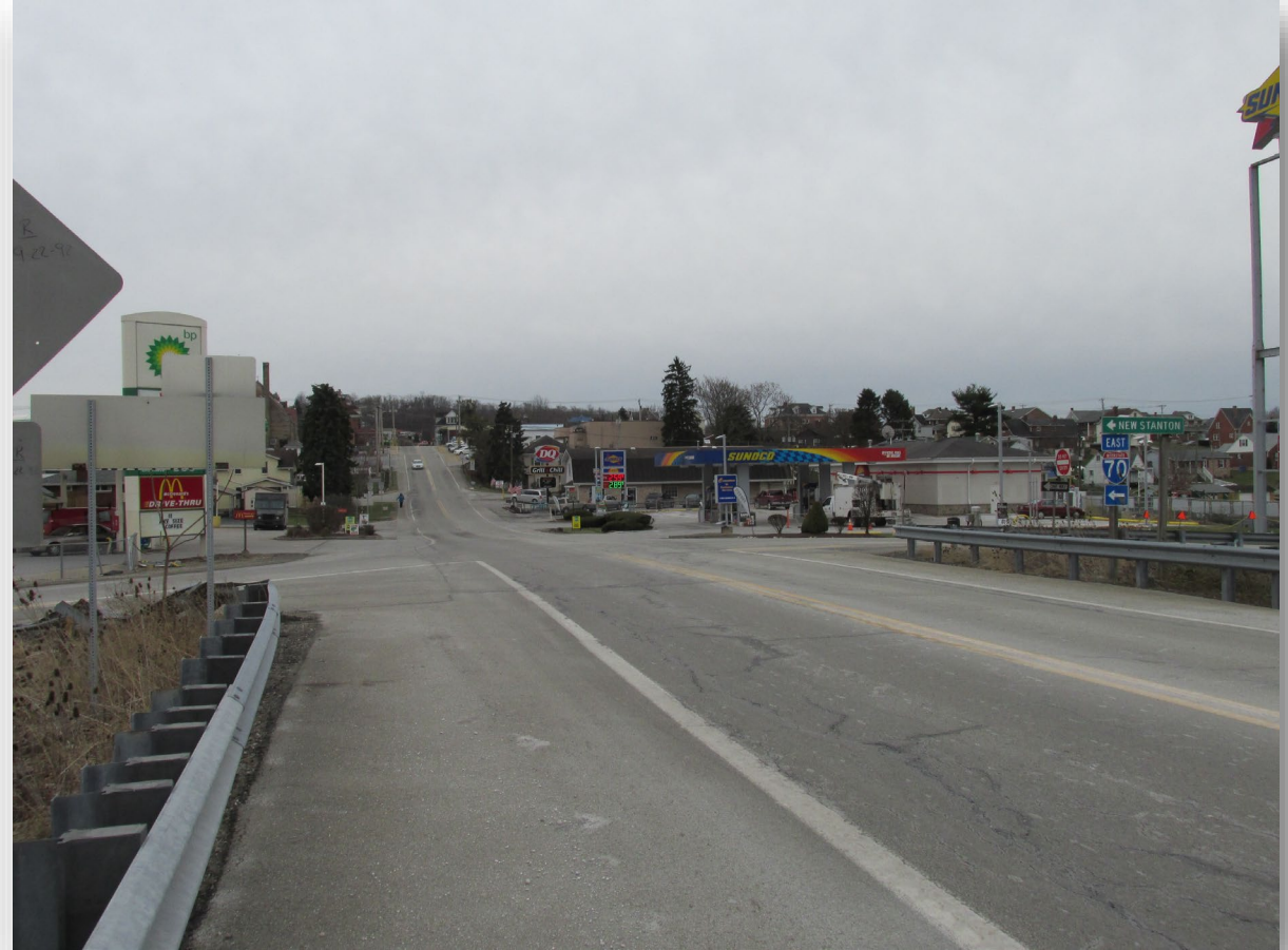
Start of Work, Looking South (Away From Bridge)
