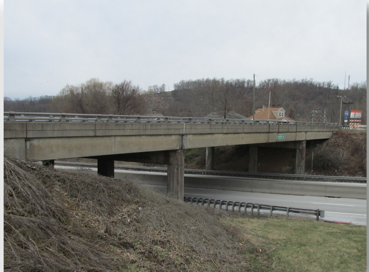
SR 3007 over I-70 (East Elevation)
