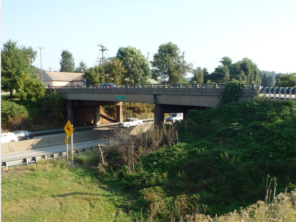
SR 3007 over I-70 (West Elevation)
