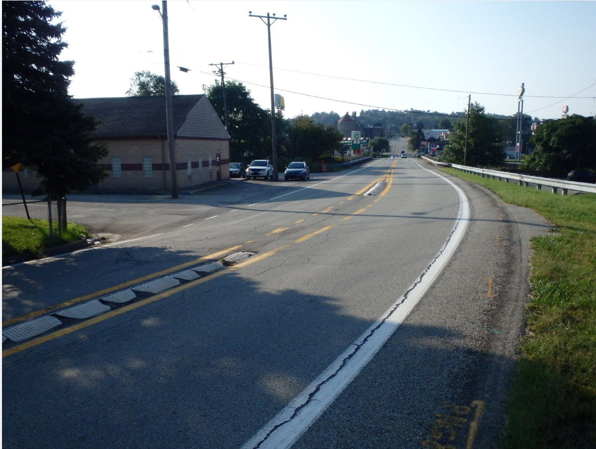
Stop Work, Looking South (Toward Bridge)
