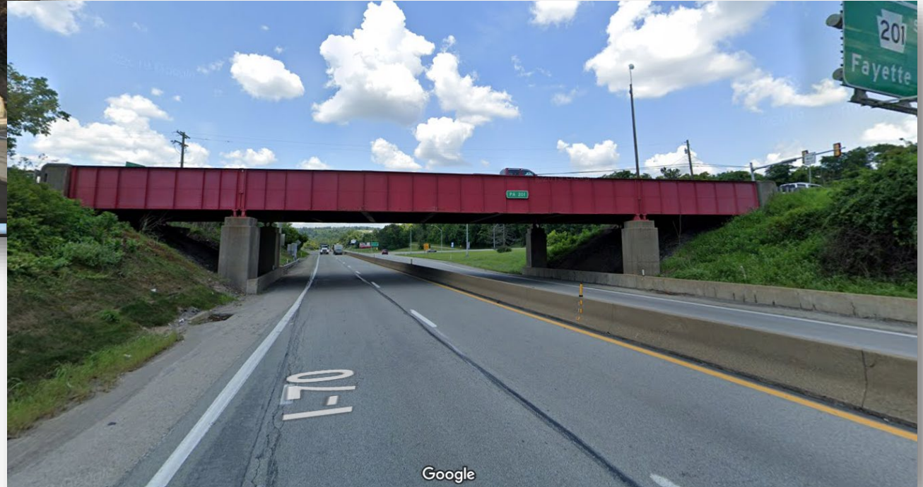
I-70 at SR 201 Bridge, Looking West
