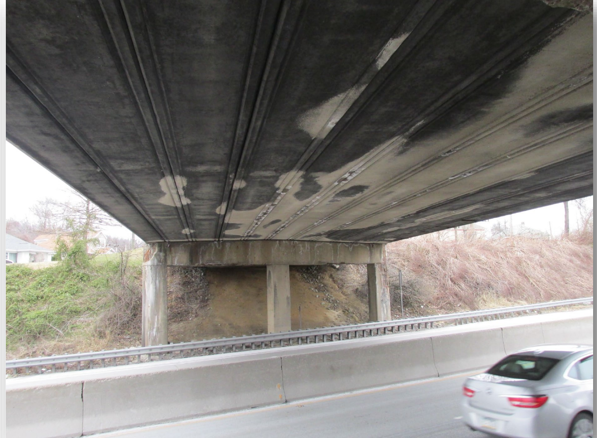
SR 3007 over I-70 Under Deck
