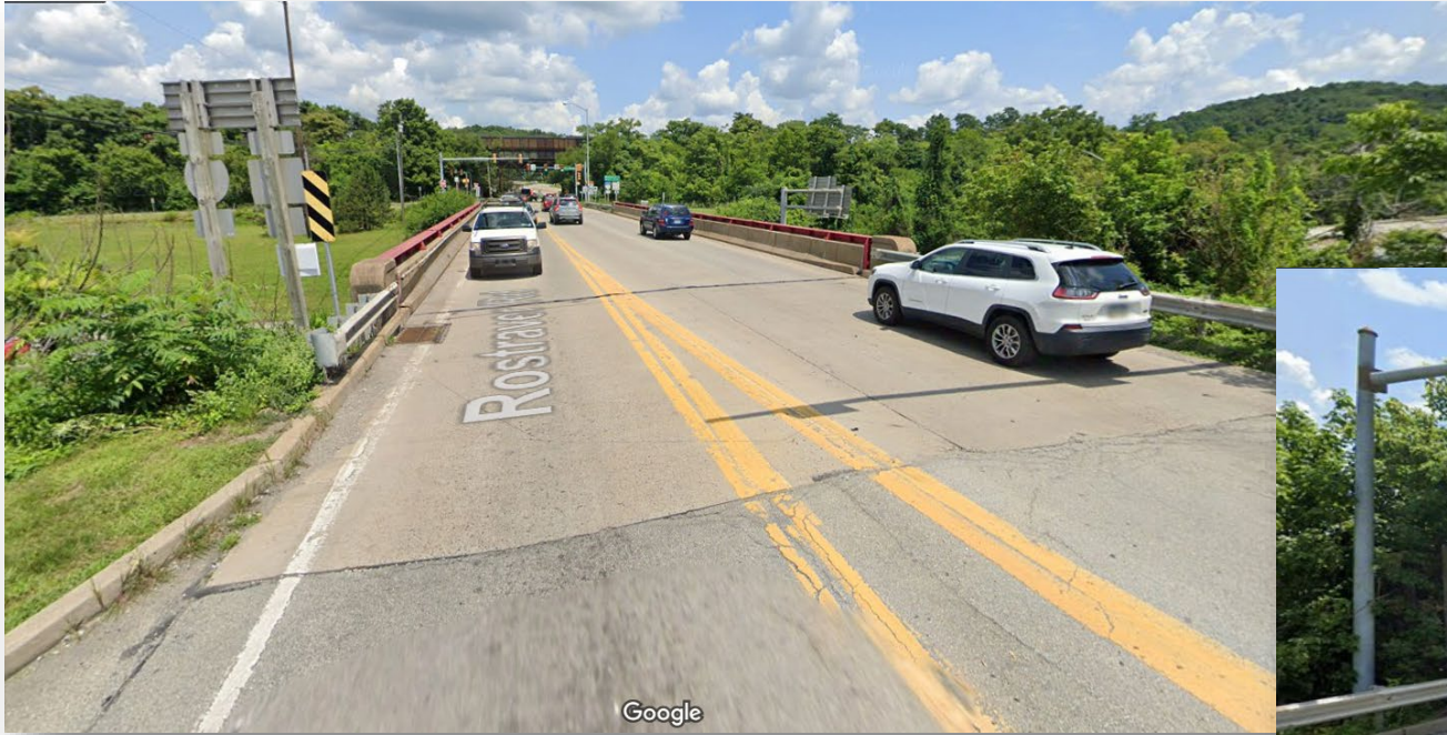
South End of SR 201 Bridge, Looking North
