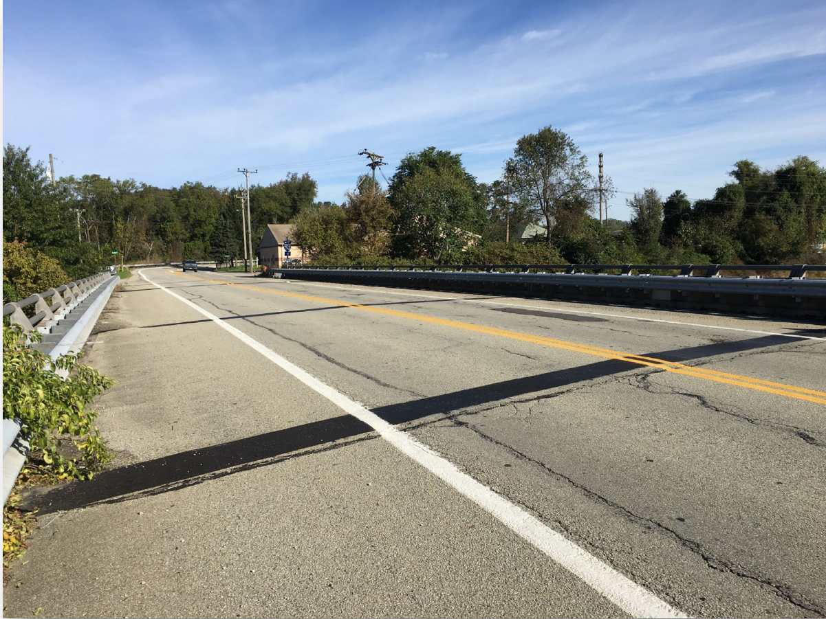
SR 3007 over I-70 Bridge Deck (Looking North)
